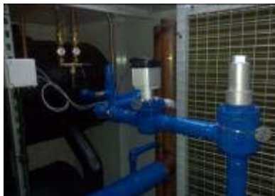
Capped stop valve to the right of the photo with the control actuator to the left
