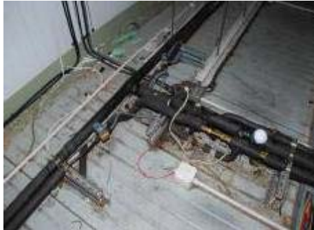
Poorly laid out pipework on the ceiling void of a chill store
