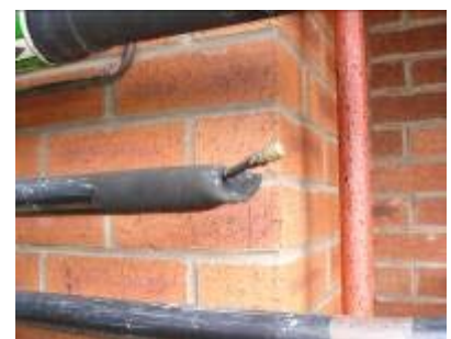
A Schrader badly fitted into the end of a poorly sealed copper pipe
